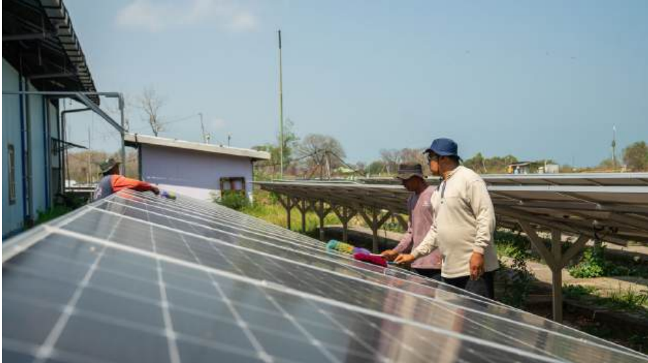
A solar-powered system converts brackish water into safe drinking water, offering a climate-resilient solution to meet the daily needs of remote communities.
