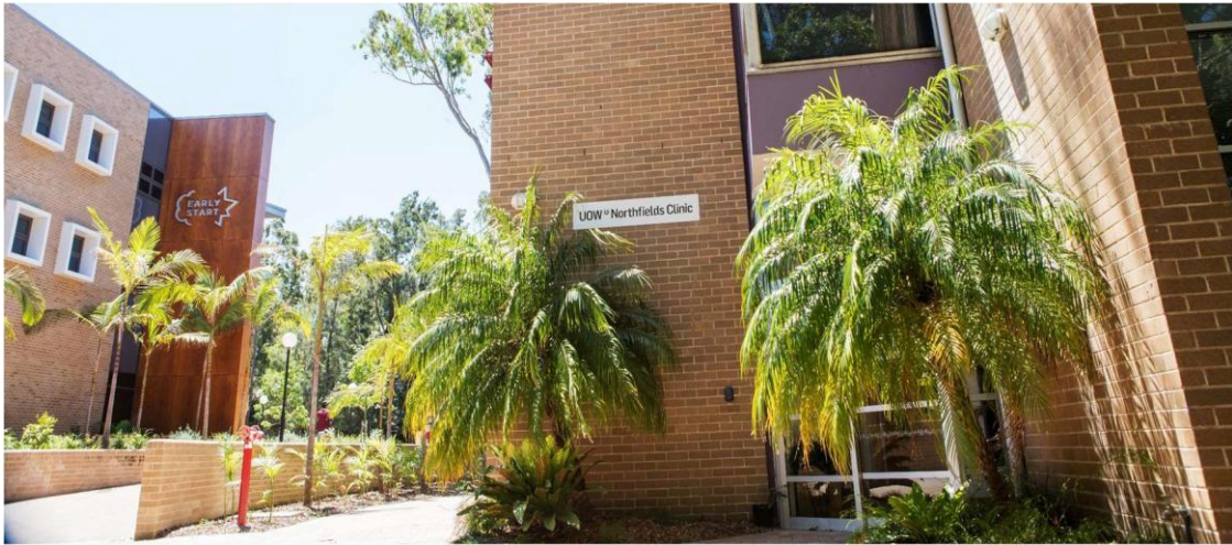
The Northfields Psychology Clinic Precinct at the University of Wollongong: Northfields Clinic@Early Start on left, Northfields Psychology Clinic, Bldg 22 on right
