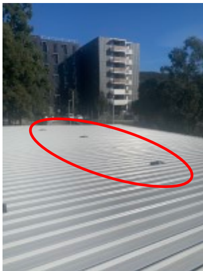
Roof area with antenna & anchors (Certification by Riverlands Roofing Status Current)
