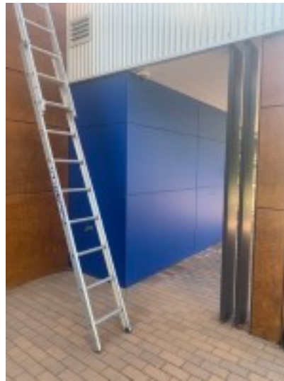
Portable ladder access
