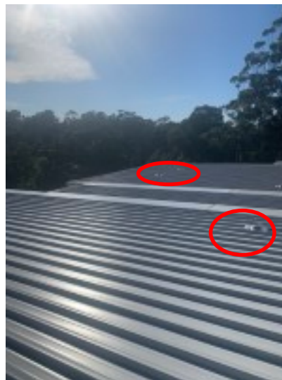
Roof area with anchors (Certification by Riverlands Roofing Status Current)
