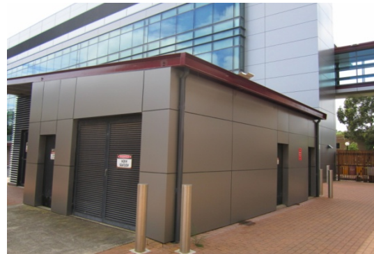
View of north west corner
