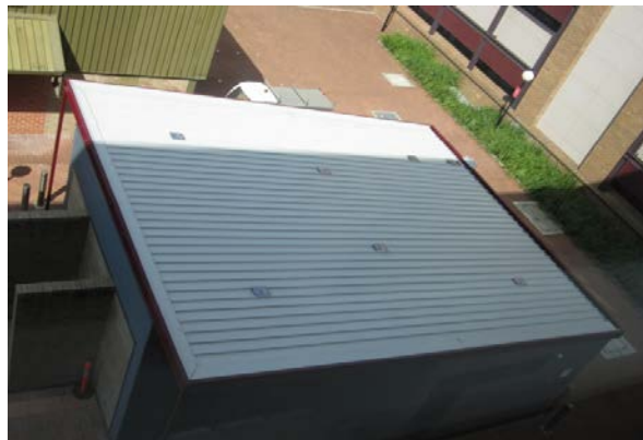
View of anchor points from Building 32
