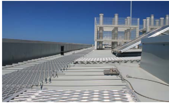
Upper roof looking north east
