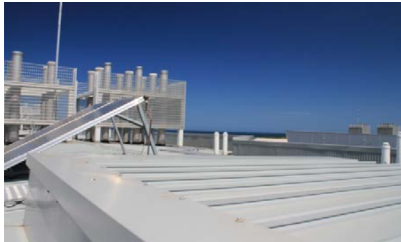
Upper roof looking south east
