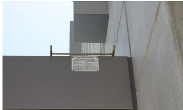
Ladder bracket to access awning
