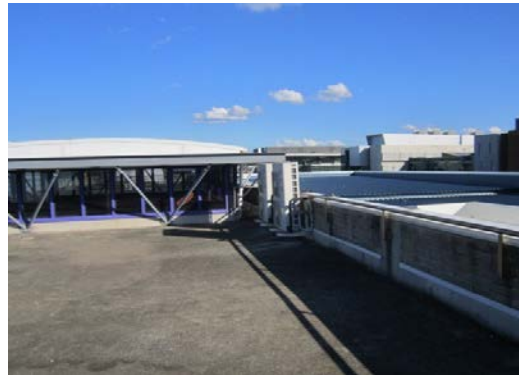
Skylight looking south
