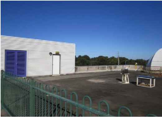
Main access door and door from plantroom onto roof
