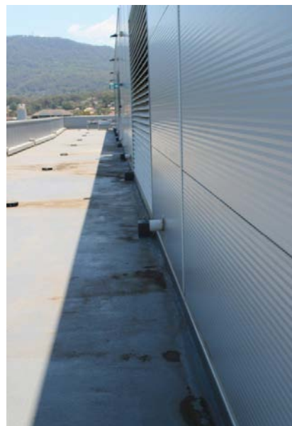
Southern side of roof
