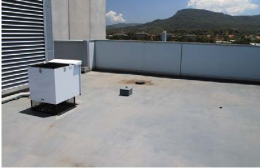
Anchor point on north west corner
