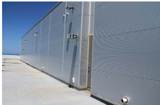
North access door from Plantroom
