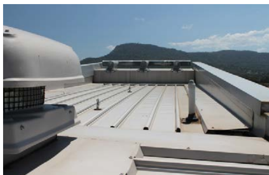
Upper roof looking west from hatch
