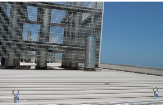
Upper roof looking east from hatch
