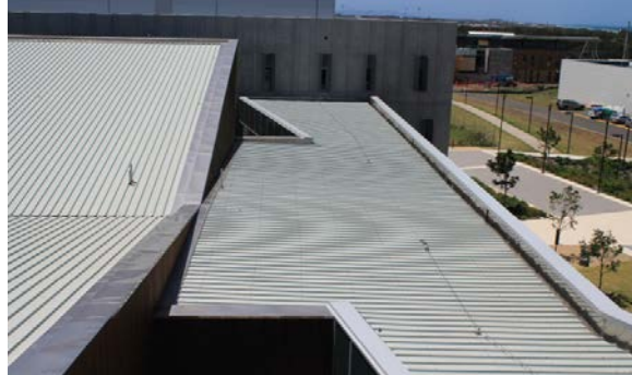
Eastern wing looking north
