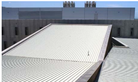
Western wing looking north
