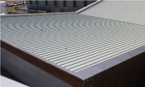
South western aspect
