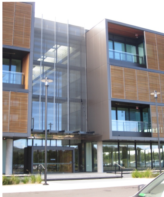
Western aspect showing horizontal lifelines used to clean windows
