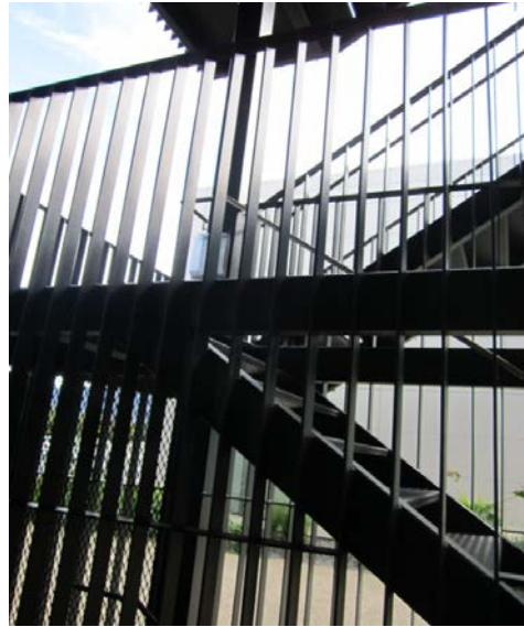
Exterior Fire Stairs requiring additional security measures
