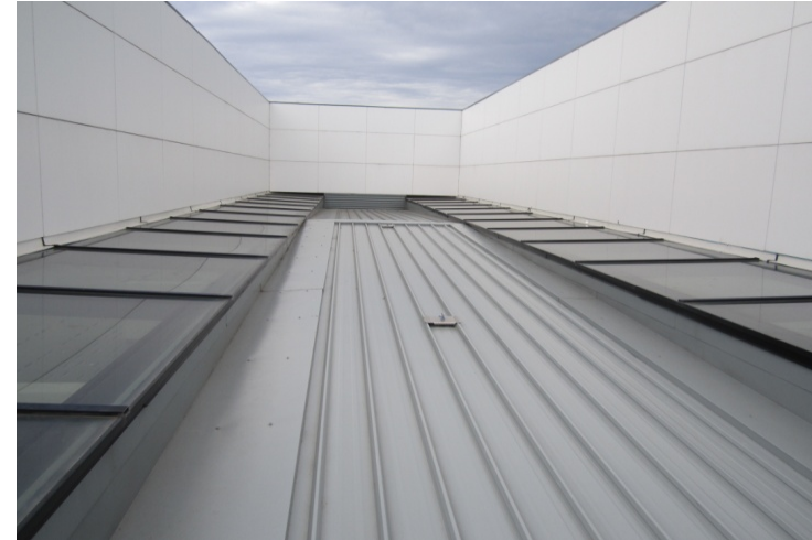
Skylights over atrium
