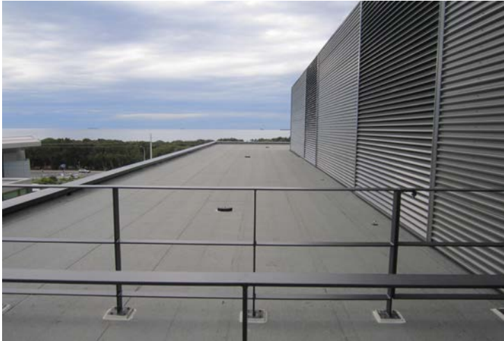
Northern roof from access looking east
