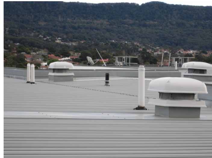
Roof over plantroom
