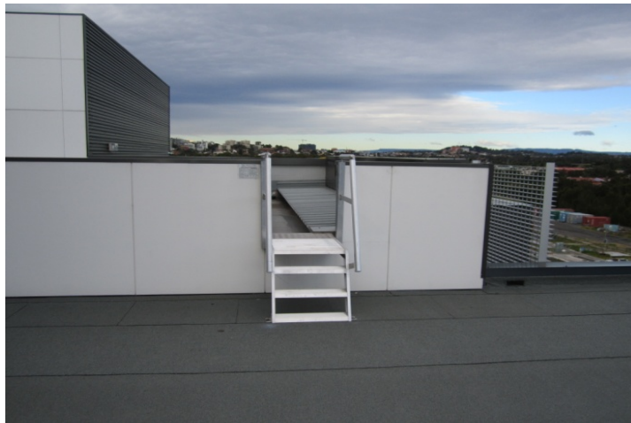
Stile to western skylights over atrium
