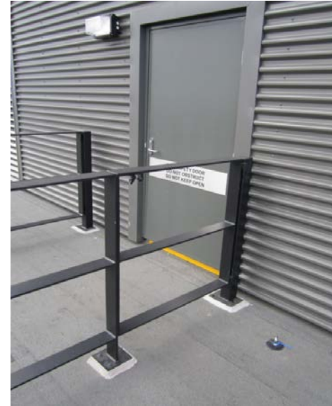
Access door from plantroom
