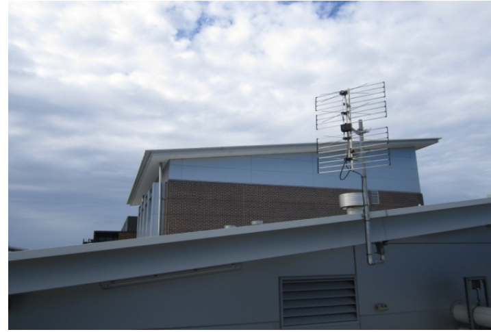
Roof over plantroom
