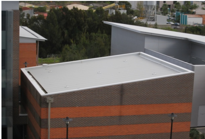
Roof of Theatre
