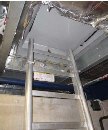
Ladder in plantroom to Western roof
