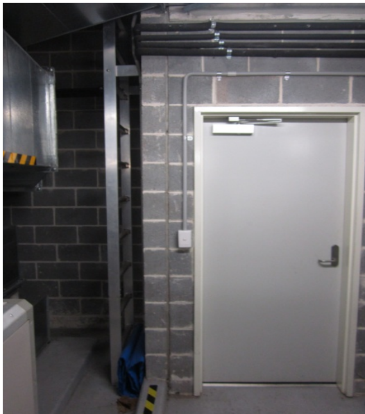
Door to plant room and ladder to roof of eastern wing
