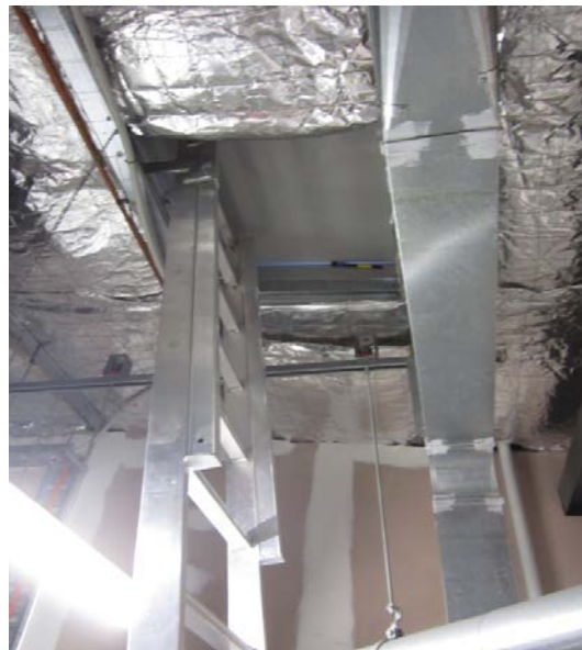
Ladder and hatch to roof of southern wing
