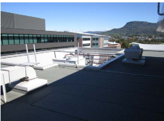
South western corner showing plantroom
