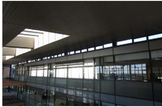
Offices in Block B under Horizontal Lifeline
