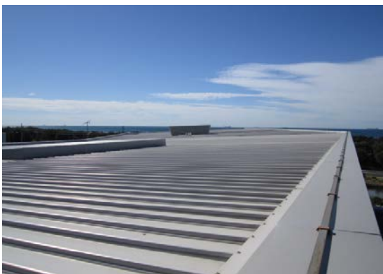
Roof of Block C looking east
