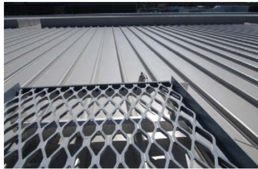
Landing from ladder to roof above atrium
