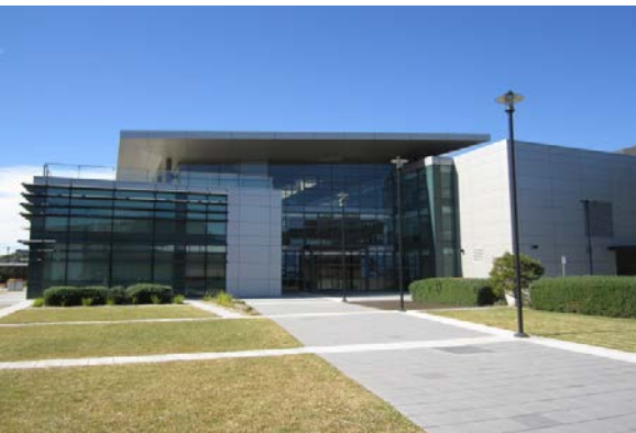
Building 230 iC Central - western aspect
