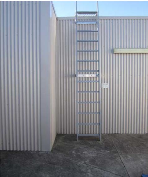
Ladder from plantroom to roof
