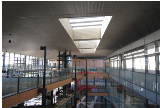
Skylight over Atrium
