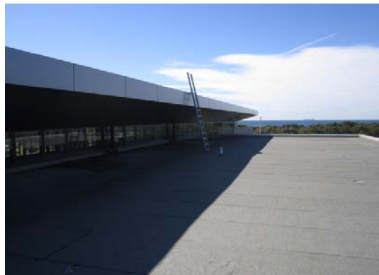
Ladder to upper roof above Block C
