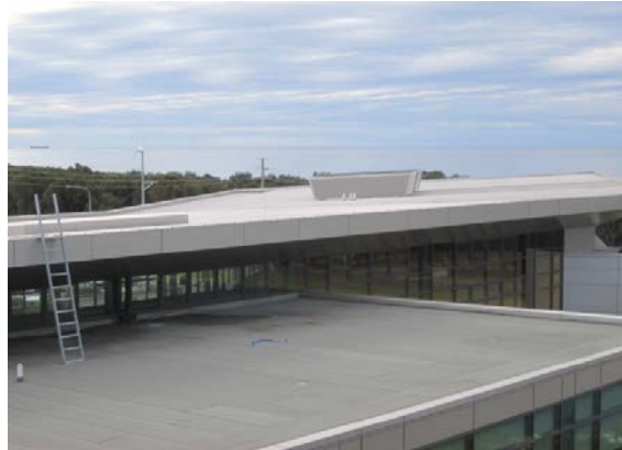
Roof over B Block showing ladder to Atrium roof
