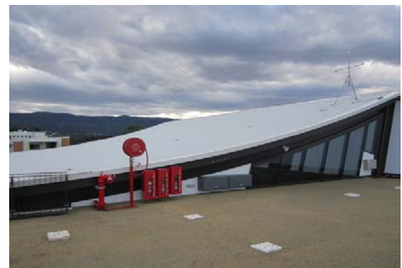
North Wing - North West aspect
