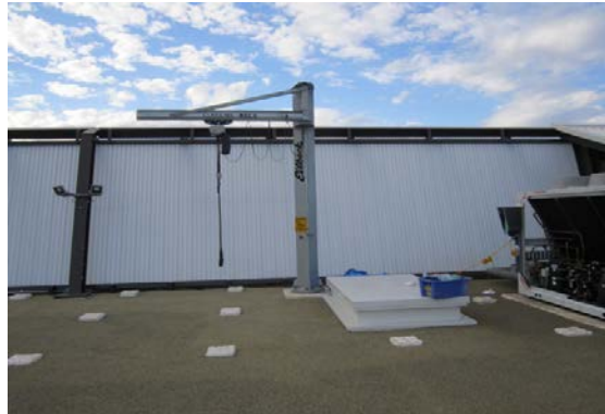
Crane and pit lid on rooftop test area
