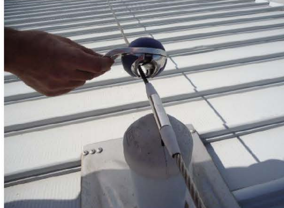
2. ATTACHMENT OF SHUTTLE
