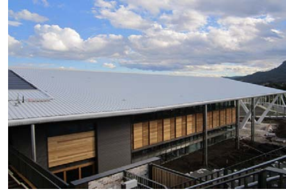
South Wing - West
