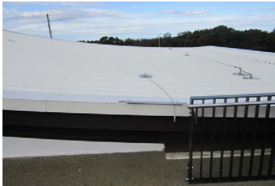
North Wing - East access
