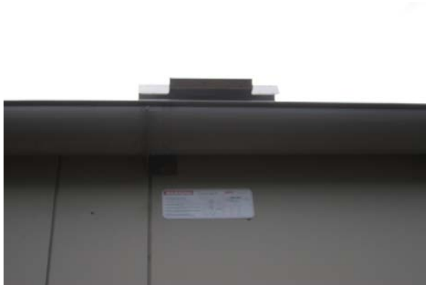
Ladder bracket on southern side
