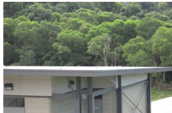
South East corner
