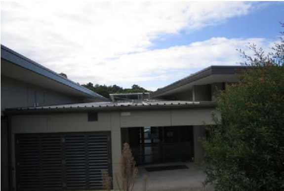
Roof access point
