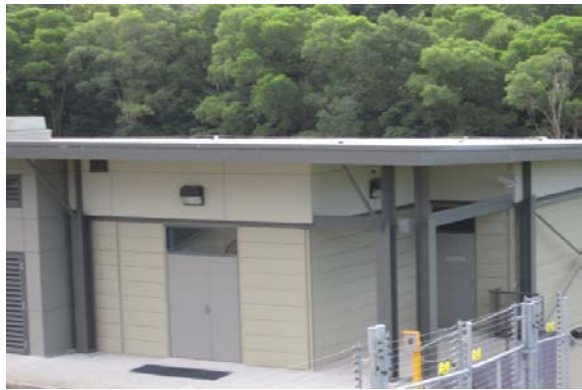
South East corner
