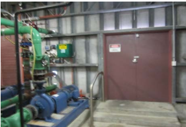
Access to roof from plantroom
