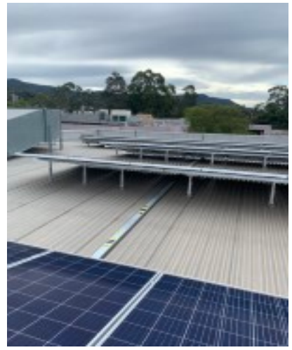
Main roof area with solar panels
