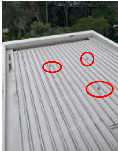
East roof with anchors (Certification by Riverlands Roofing Status Current)
