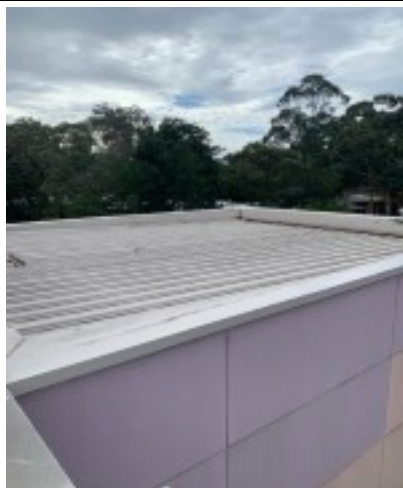
Main roof area
