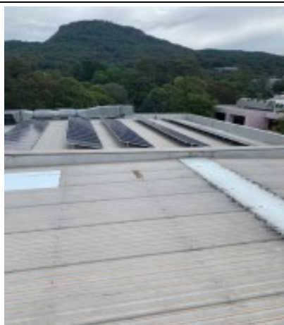
Upper roof area
