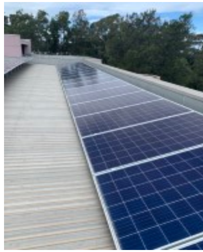
Main roof area with solar panels
