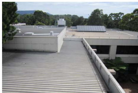
Block A looking north from ladder
