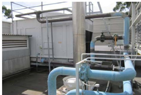
Enclosed services area in SW corner of Block C
