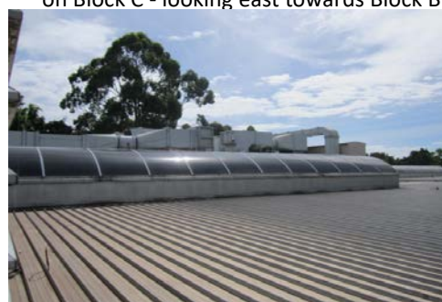
Skylight on Block C
