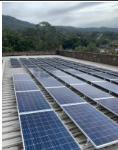
Main Roof area with solar panels
