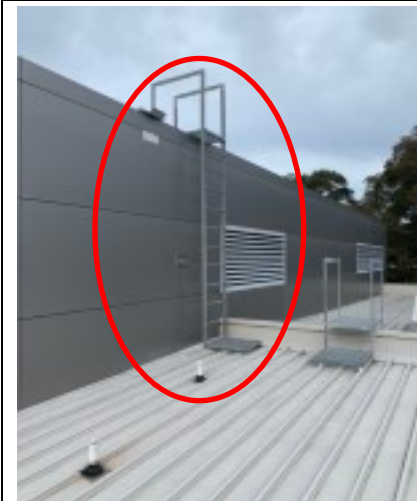
Upper roof fixed access ladder
