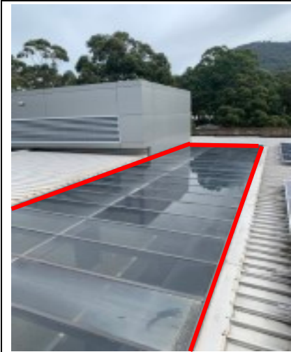
Main roof area Caution Glass Skylight do not walk on glass
