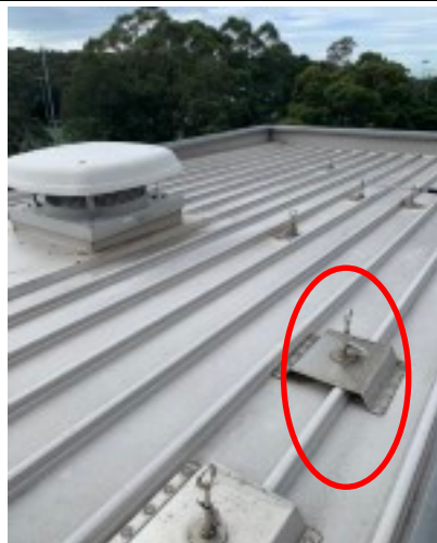
Upper roof area with anchors ( Certification by Riverlands Roofing Status Current )
