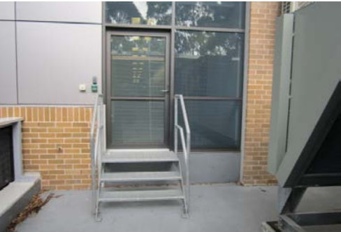
Access from Building 24 to landing
