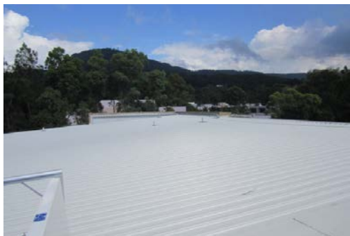
North western corner
