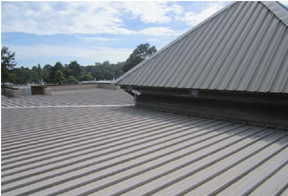
Fall restraint system around the pyramid skylight
