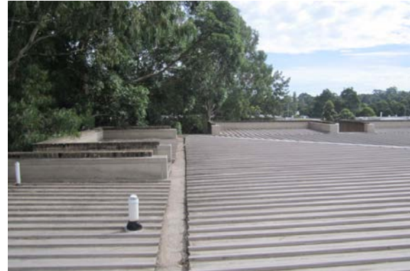
View North-West corner
