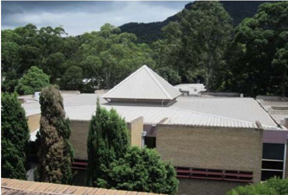
View of Eastern aspect from Building 67
