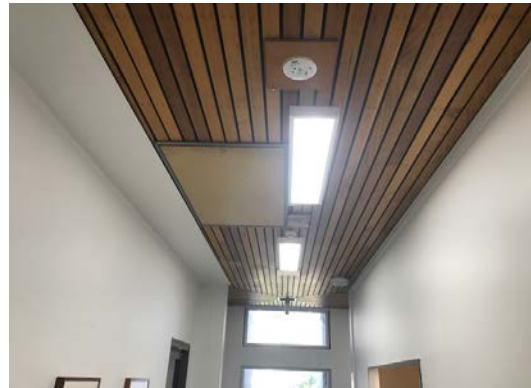
B22 roof cavity fold down ladder
