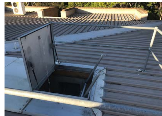
B22 roof access hatch
