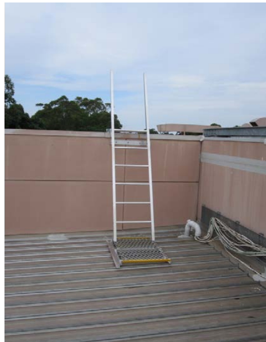
Ladder to access Building 11
