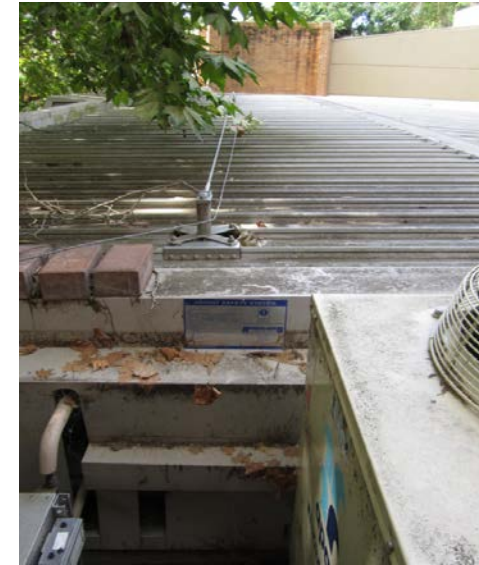
Location of compliance plate south east annex
