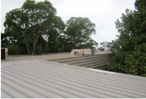
Northern wing - eastern view
