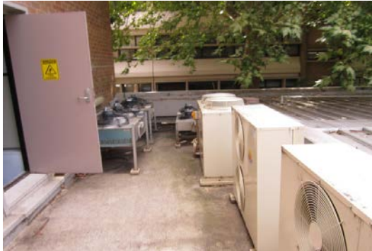
Access to south east annex landing
