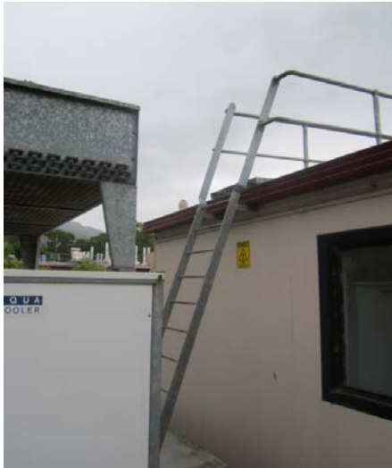
Ladder to access Northern wing
