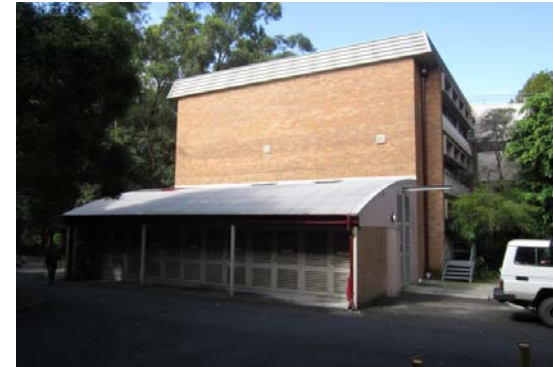
Gas storage annex on western side of Building 15
