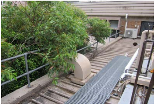
Walkway behind plantroom
