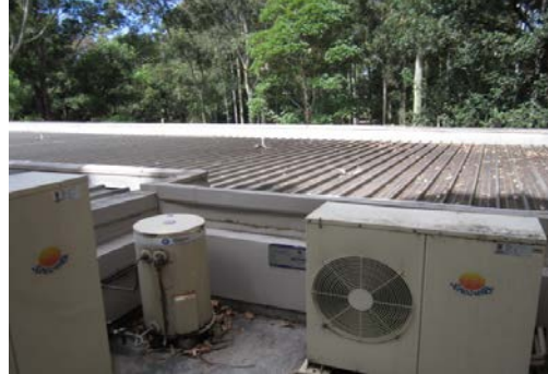
Location of compliance plate south east annex
