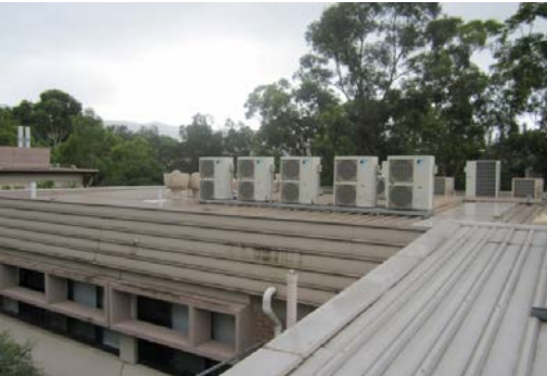
Northern wing - western view
