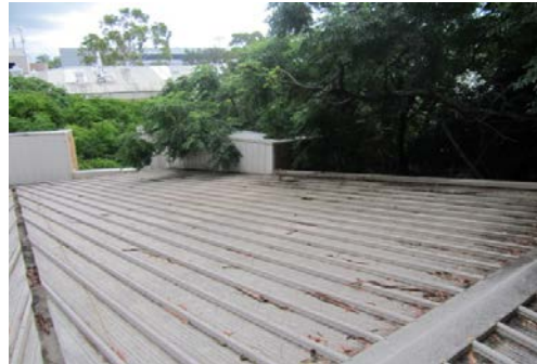
Main Roof over Lecture theatre looking north east towards Building 35
