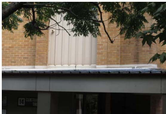
Awning over front of Building 14
