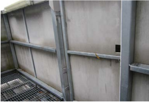
Gate from landing onto roof proper
