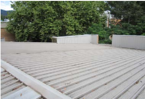
Main Roof over Lecture theatre looking north west towards Building 15
