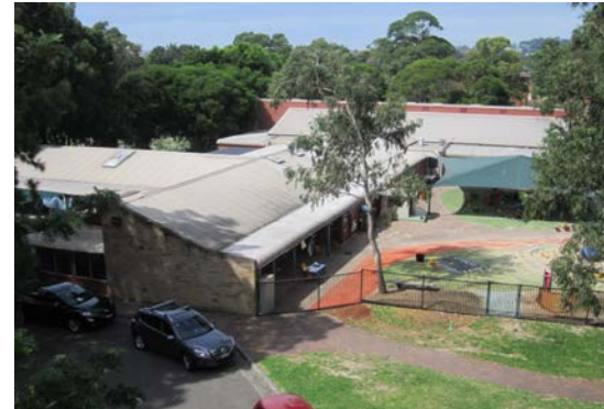
View of roofs from Building 39
