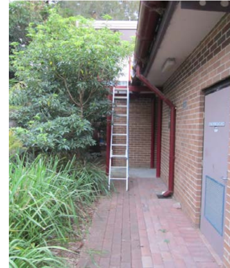
Temporary ladder access to roof
