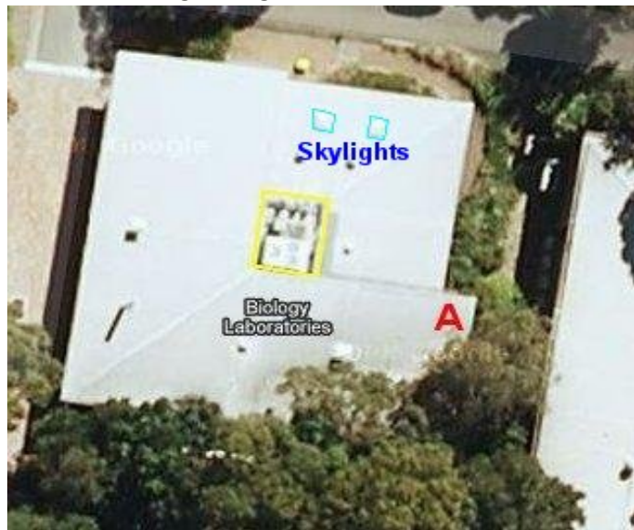
A - location of access to roof (ladder bracket) _____ Safe Roof Work Area
