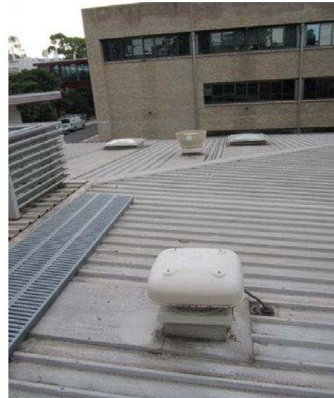
Looking north towards skylights
