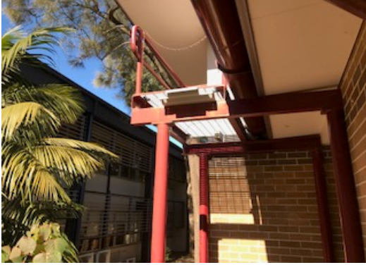
B5 roof access ladder bracket
