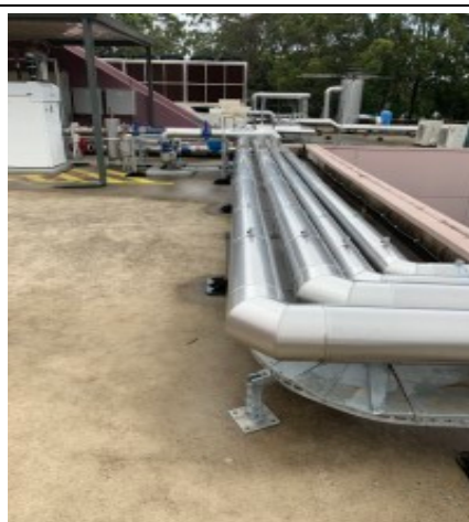
Building 3 roof area with exposed pipework
