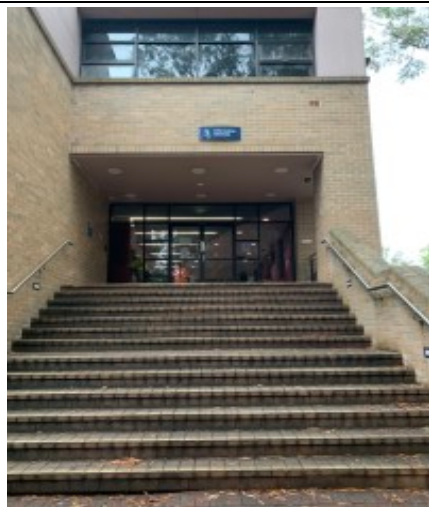
Building 3 entry steps
