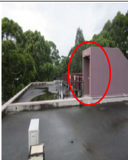
Building 3 roof access door and roof area
