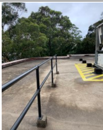
Building 3 roof area
