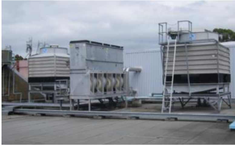
Figure 8: Cooling towers
